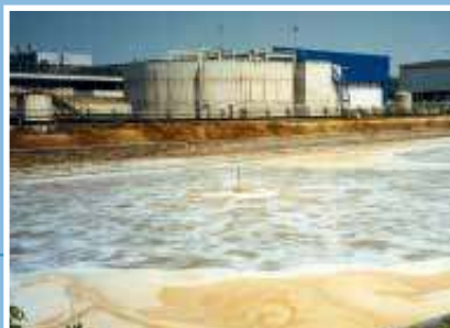
Aeratori sommersi tipo SCL installati in impianto di depurazione. Submersible aerators type SCL installed in a wastewater treatment plant
