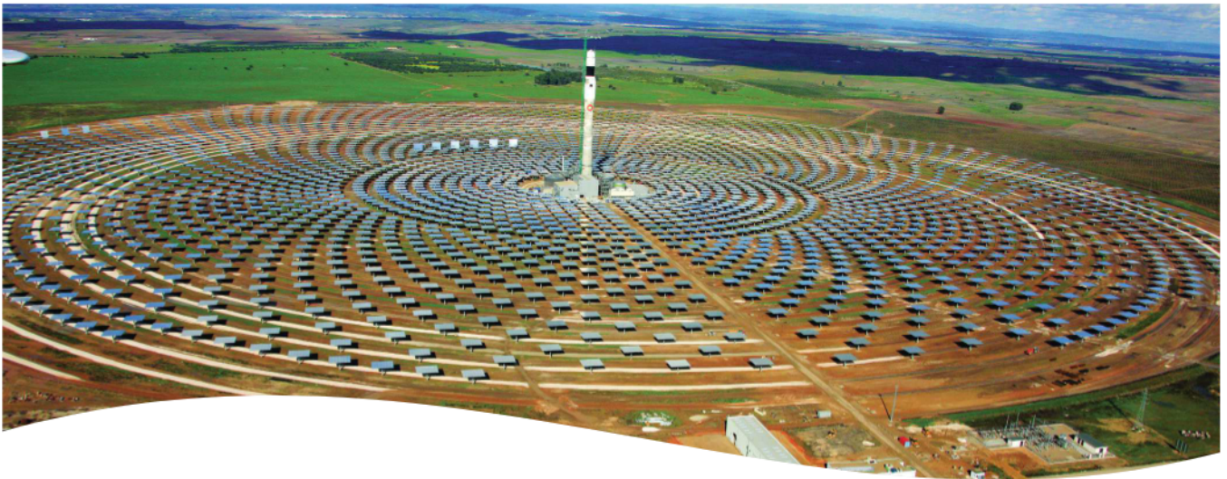
Gemasolar plant. Property of Torresol Energy. © Torresol Energy
